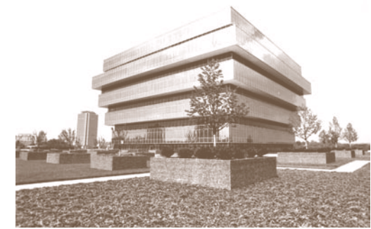
The GTE building as it is today: "Little in common with the formal language of Bisharat's original master plan."
